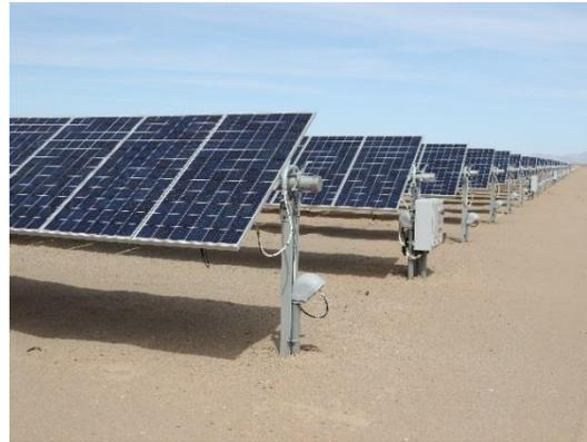
The tracking system would be supported, when practical, by driven piers (piles) directly embedded into the ground and would be parallel to the ground. The system would rotate slowly throughout the day at a range of +/- 60 degrees facing east to west to stay perpendicular to the incoming solar rays so that production would be optimized.
